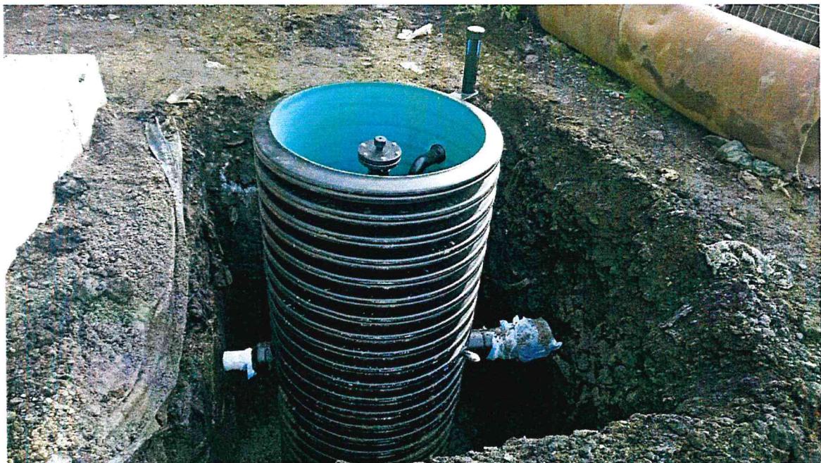
Figura 9 Camin condensat preechipat instalat in lucrari similare
